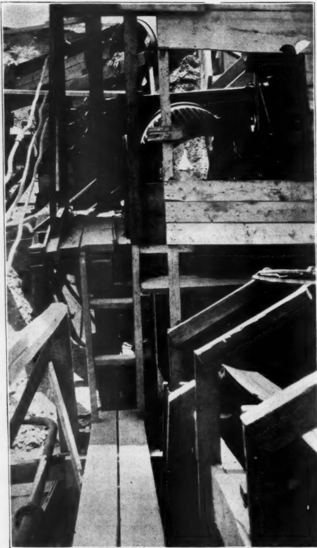
Conveyor Discharging into Scalping Screen. Right Foreground Conveyor to Sizing Screens
